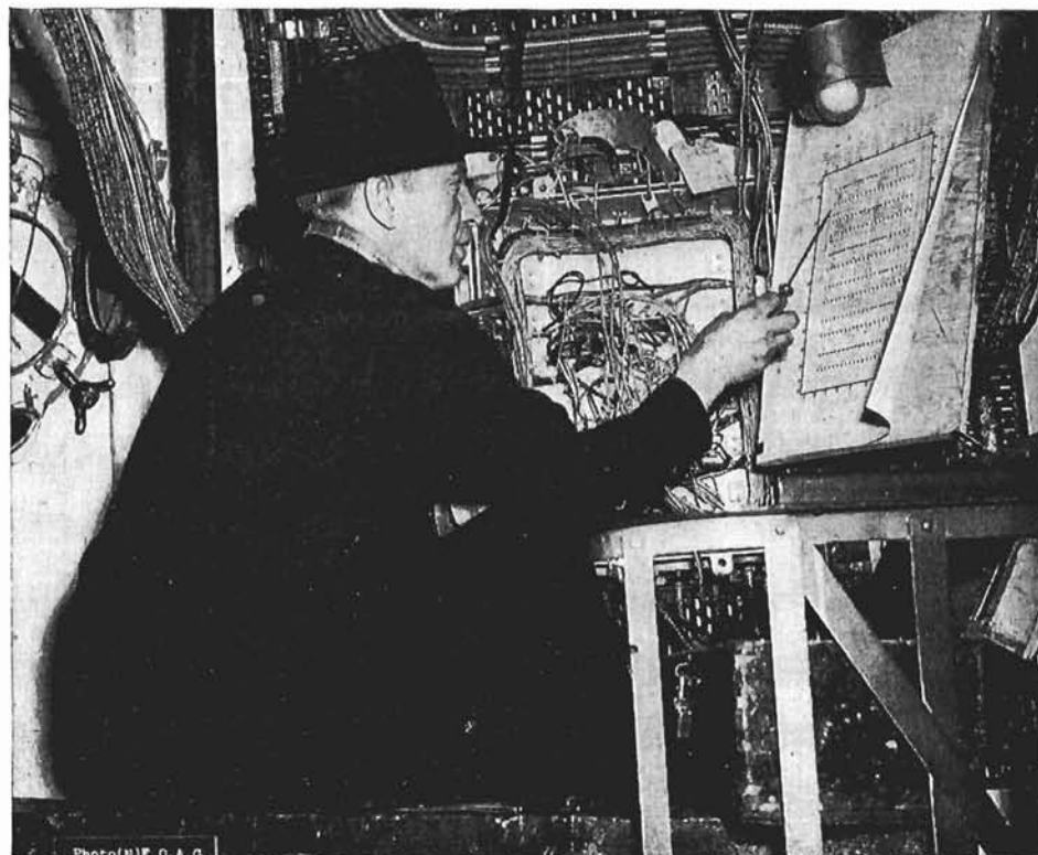
Electrical Journeyman Dean Wood gets set to connect the mass of wiring in a newly installed junction box in HMCS "Nootka". Mr. Wood is one of a crew of 30 civilian electricians engaged in the conversion of the "Nootka". (HS-10711.)
